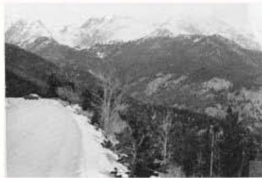
Rural roadside hazard rating of 7.
