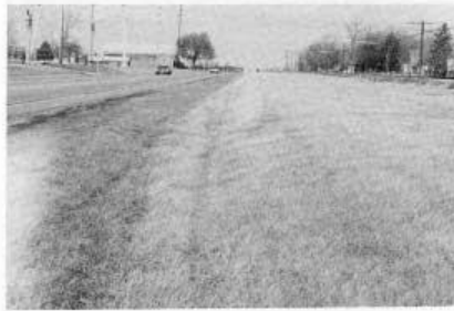
Rural roadside hazard rating of 1.
