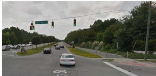
Figure 6 Protective-permissive left turn signals may be confusing to pedestrians attempting to rely on the vehicular traffic signals to know when it is their turn to cross, and therefore engineering judgement must determine whether Section 1.3.2.1 D of the 2009 MUTCD applies.
