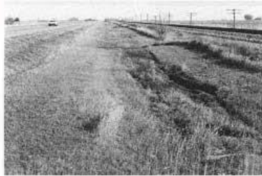
Rural roadside hazard rating of 2.
